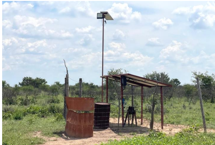
Plate 1-8 Example of a borehole extracting underground water using either a solar power system (as in this case) or a fuel-powered engine.
