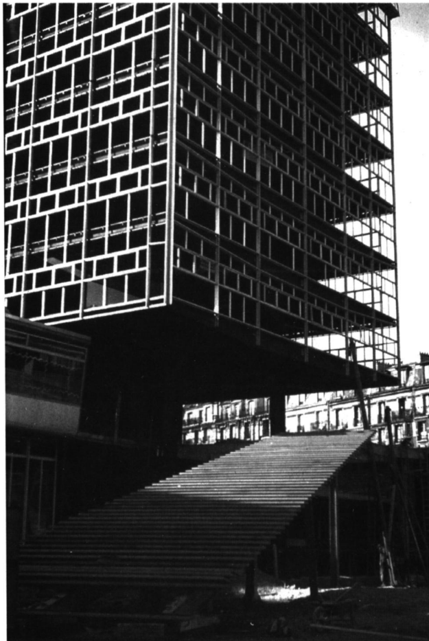
Figure 8. CAF, Wallspan grid during assembly. Photo Henri Longepierre. Archives privées Henri Longepierre.
