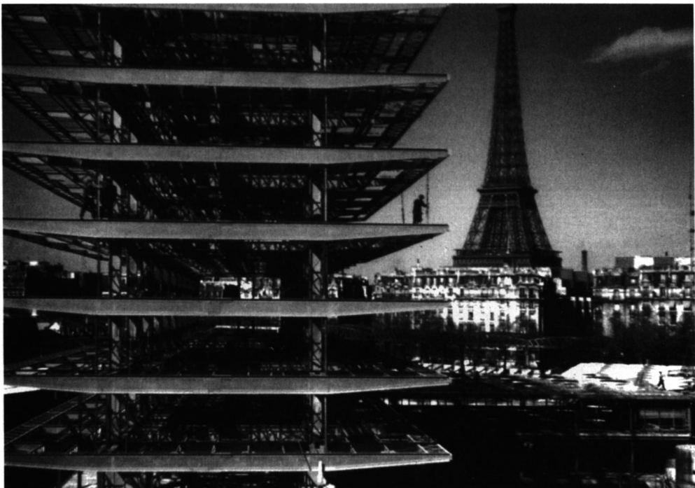
Figure 3. CAF, steel frame during erection, 1957. Photo Henri Longepierre. Archives privées Henri Longepierre.
