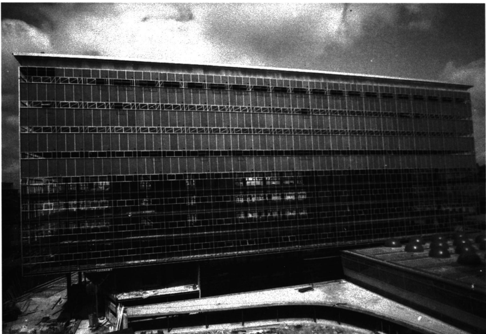
Figure 10. CAF, Wallspan grid and Héliotrex panels during installation. ACAF.
