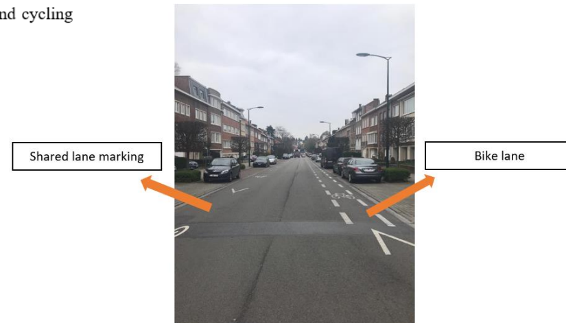
Fig. 3 The different cycling infrastructure types on the road used for the cycling trips
