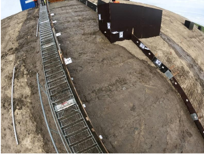
Figure 4. Test section for the lime-treated clay tests
