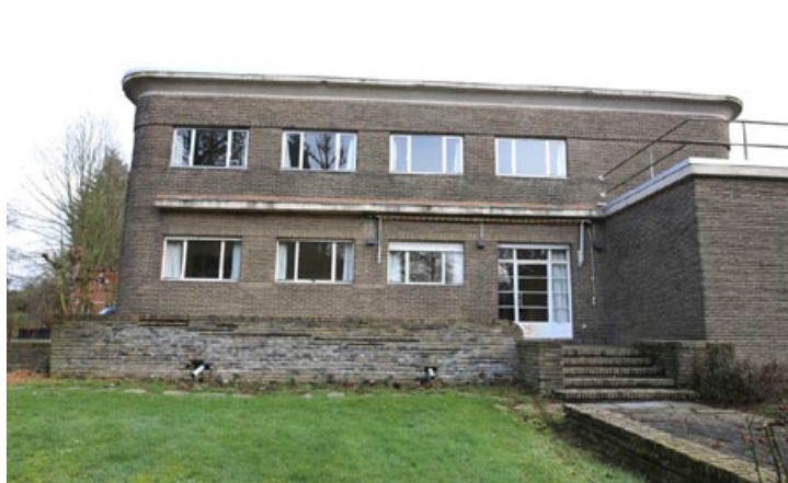
Figure 4. Building B: a case study in Tervuren. Photo: Samuel Dubois.
