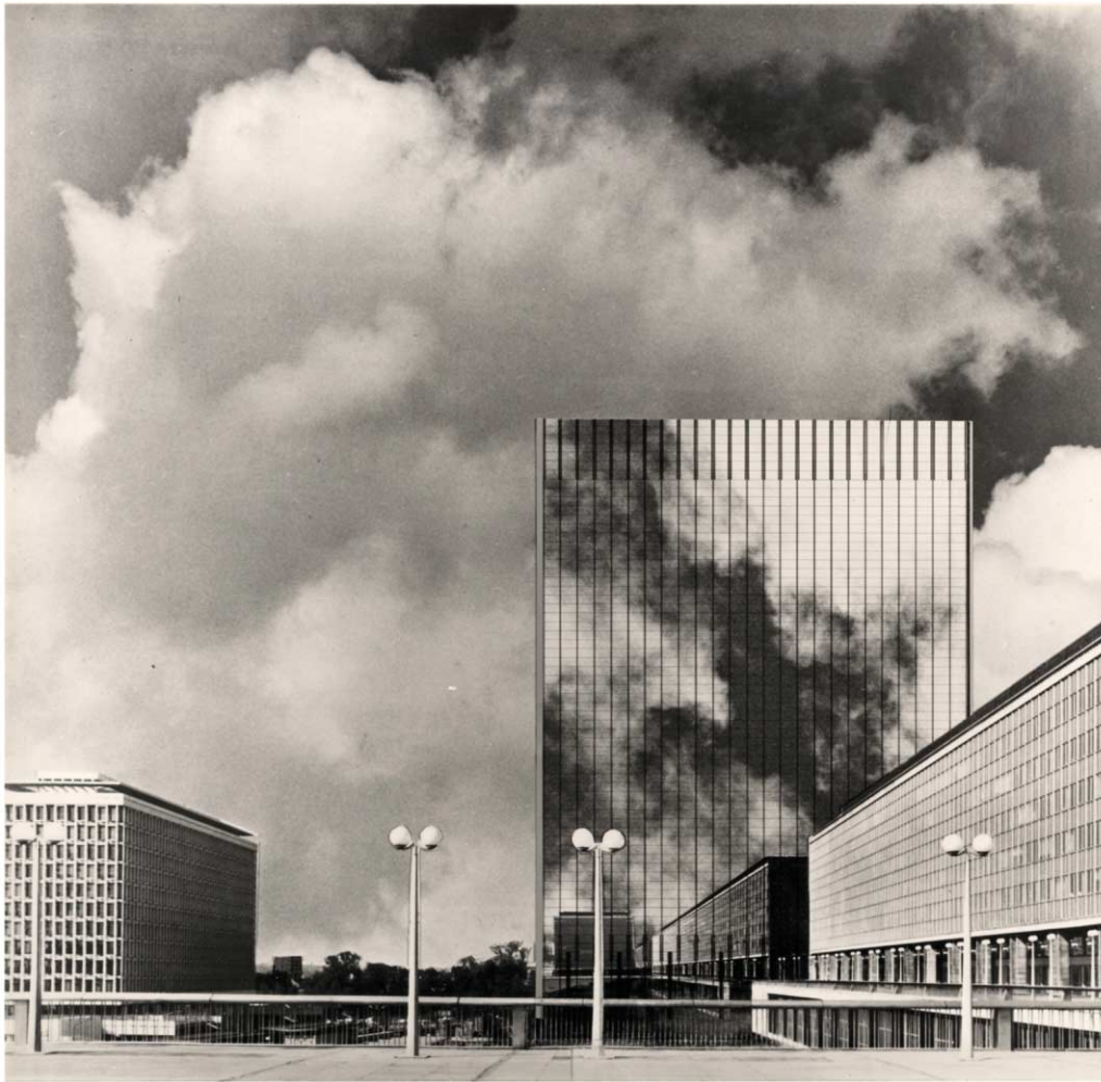
Figure 5. The CAE site in 1984. Source: Archives d'Architecture Moderne, Bruxelles.
