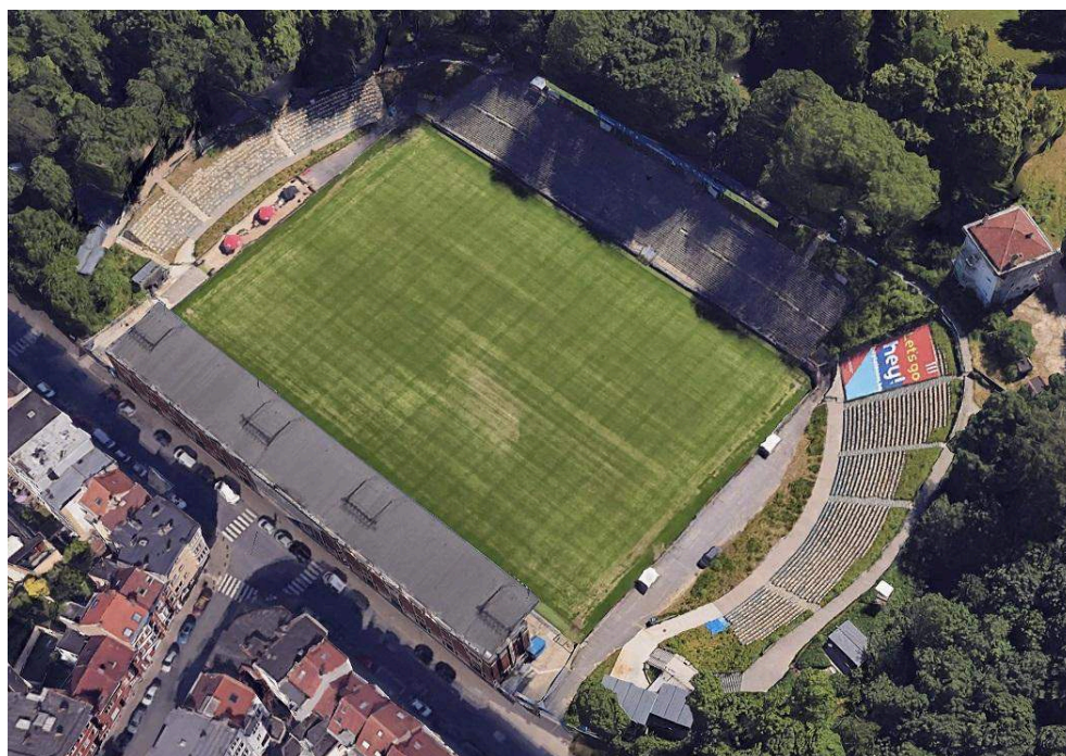
Figure 1. View of the current stadium: Stade Marien
