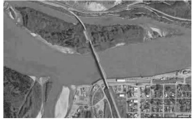
Figure 6. Aerial view of the Parks Highway Bridge over the Tanana River, Nenana, Alaska, US (Map: Google, Digital-Globe 2017).
