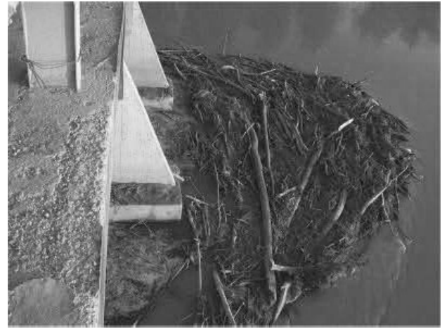
Figure 2. Clogging phenomenon on a bridge over the Po River, Guastalla, Italy (Malerba, et al. 2013).
