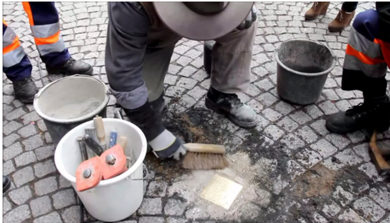
Re-laying the Original Stolperstein. Köln, Germany. 2013.
