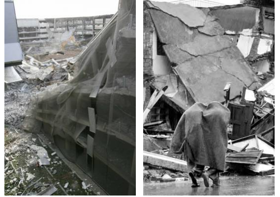
Fig. 5. Two typical non-parallel slab-based structures.
