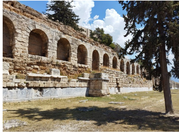
Fig. 2. Current state of the remains of the Stoa of Eumenes II, showing the arched retaining wall and part of the rear wall.
