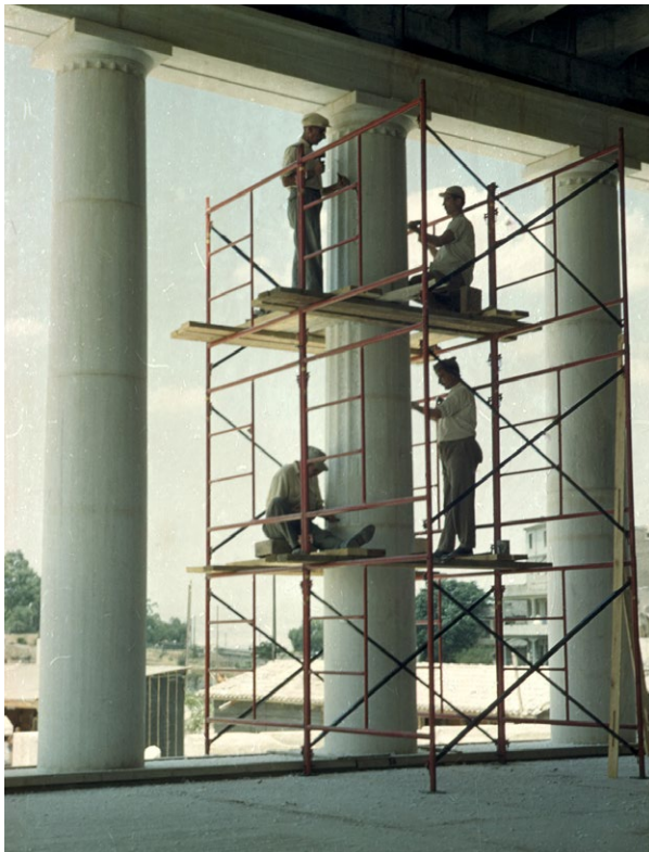
Fig. 7. Fluting the first Doric column during the restoration of the Stoa of Attalos (ASCSA, Agora Excavations).
