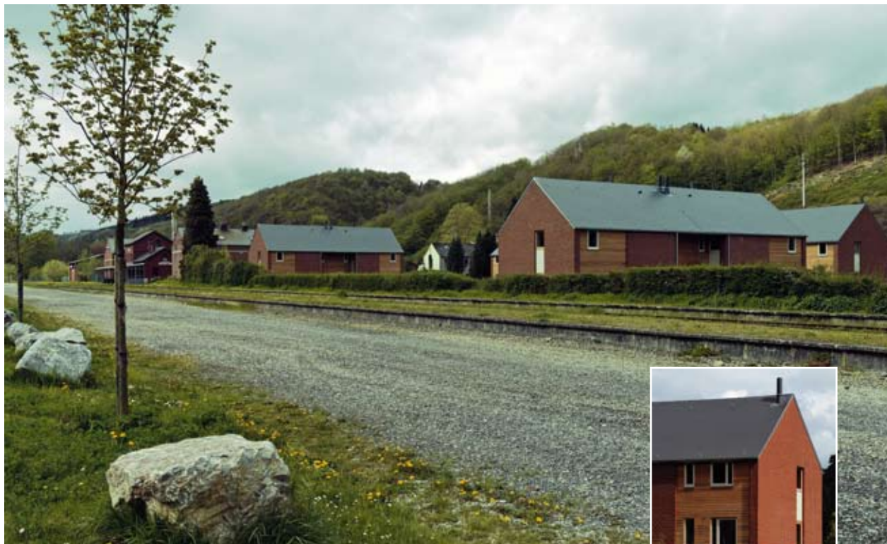
Photo : J.-C. Carpentier © SPW
