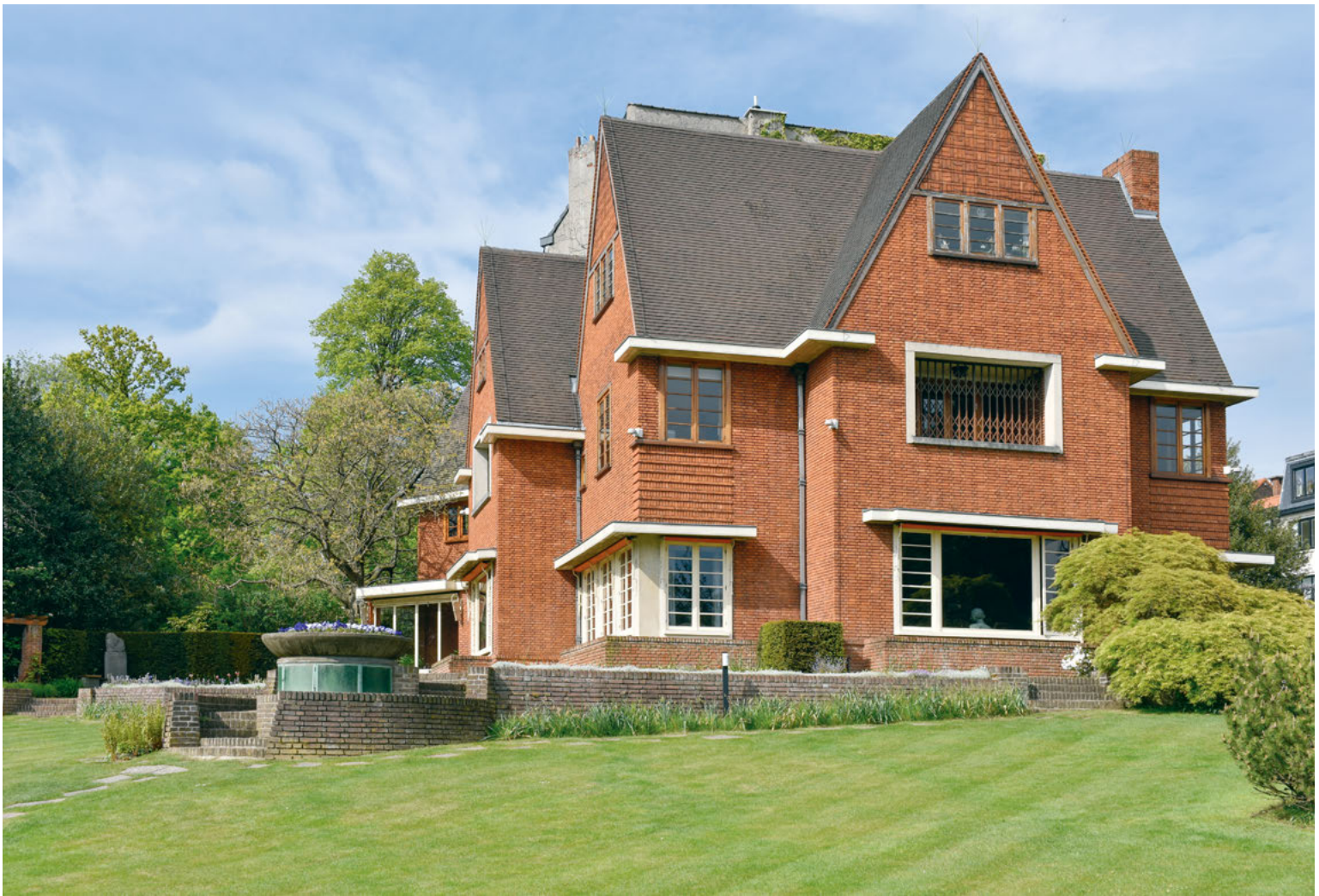
Standing alone in its private park, the Van Buuren Villa is free from terraced housing's party walls, opening up the urban block (Govaerts-Van Vaerenbergh, 1928).
