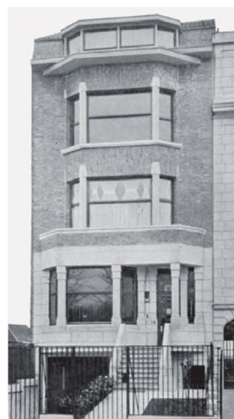
After the First World War, houses were set back from the street to allow access to garages set in sunken basements (De Ridder, boulevard Saint-Michel 97, 1923).
