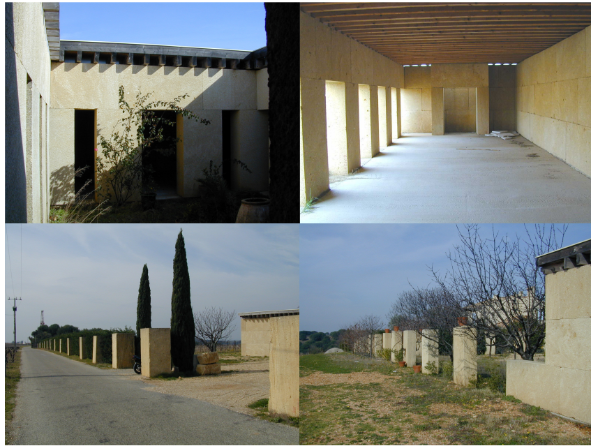
Chai Viticole, Gilles Perraudin, Vauvert, France.
