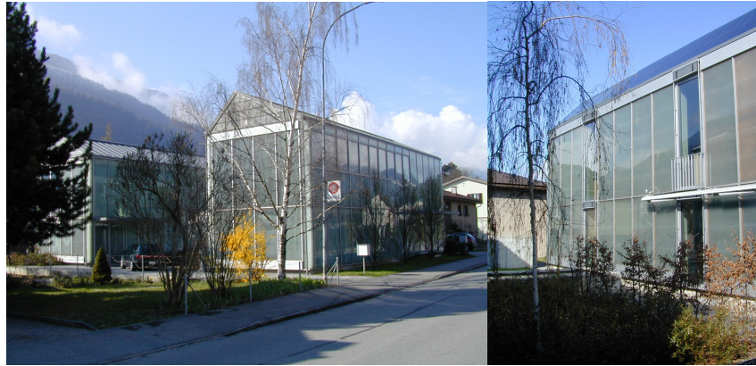
Nullenergie House, Chur, Switzerland – Isolation transparente.
