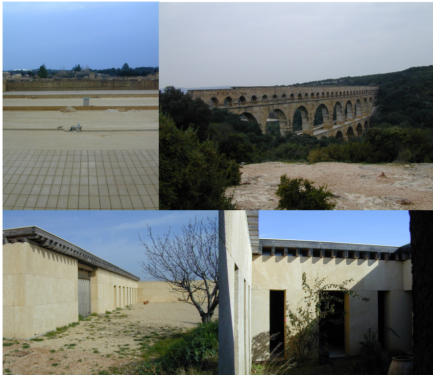
Chai Viticole, Gilles Perraudin, Vauvert, France.
