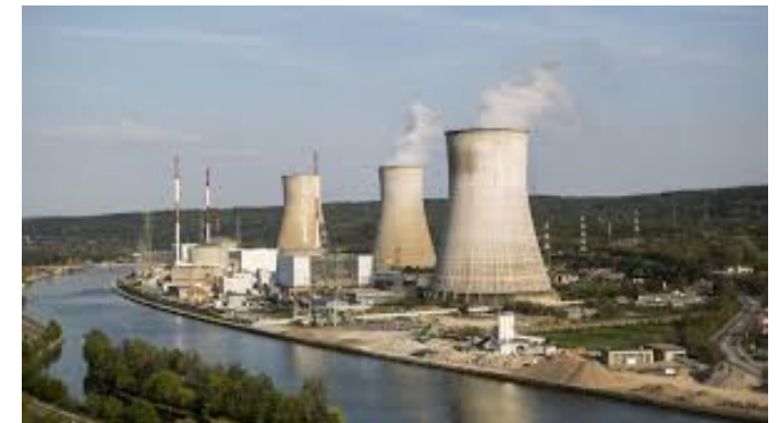
Tihange Nuclear power plant
