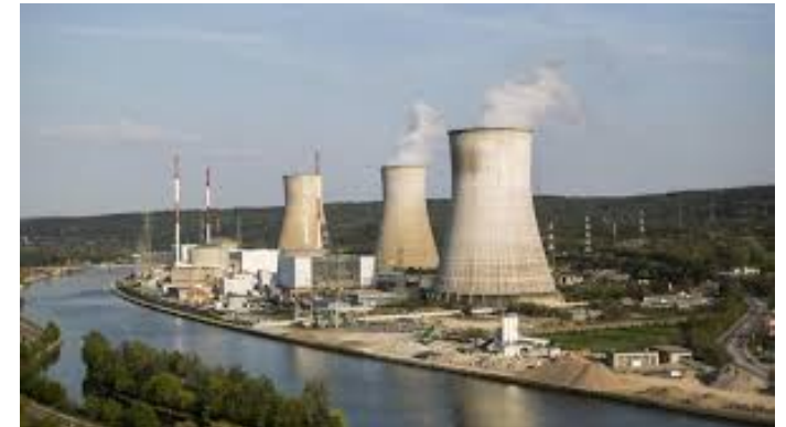
Tihange Nuclear power plant
