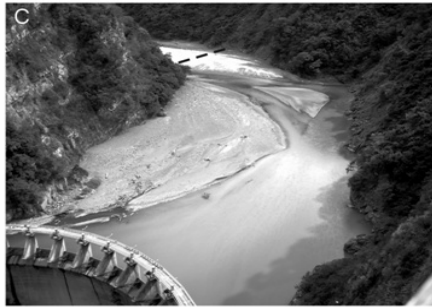
Figure 1.3: Delta front prograding into standing water: Ronghua Dam, Northern Taiwan, November 2005(photo by A.T.H. Perng). The dashed line in the background shows the location of the delta front in August 2004
