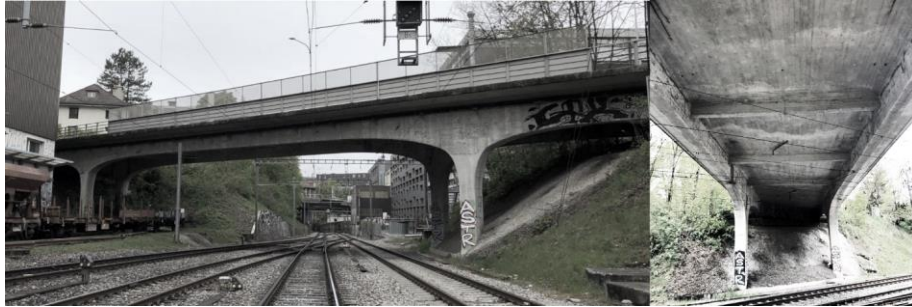
Fig. 1. the views of the Weissensteinstrasse Overpass from the east and below (photographed respectively by Maryam Jafari and Shuyuan Han in 2022)
