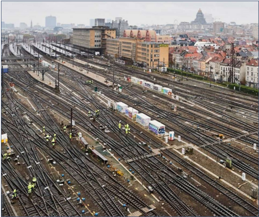
Fig. 1.1 Works of maintenance in Brussels-Midi station over a public holiday weekend: replacement of 170 switch motors to enhance infrastructure reliability and safety Source: Infrabel, Annual Report 2019 [2].
