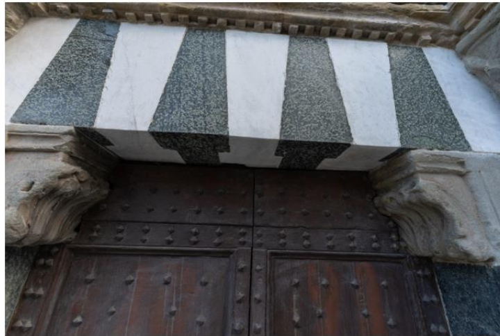
Figure 2: The flat arch crowning the transept portal in the Prato Cathedral (Photo: courtesy of Piacenti S.p.a. ).
