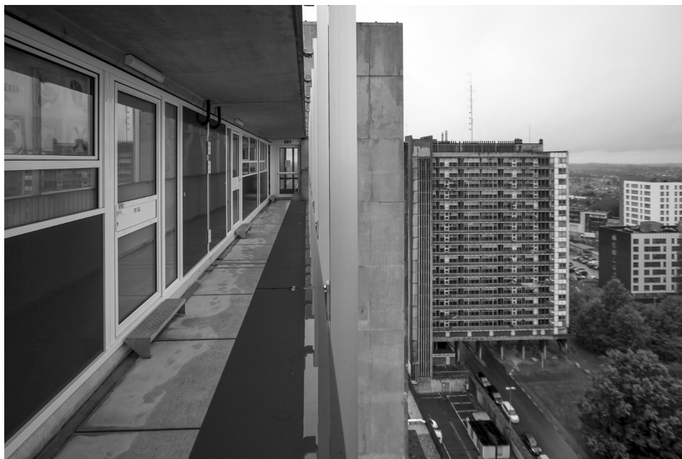
Fig. 17. View of the new joinery units on the open-air gallery of the newly renovated tower II; Alexandre Bossard 2023.
