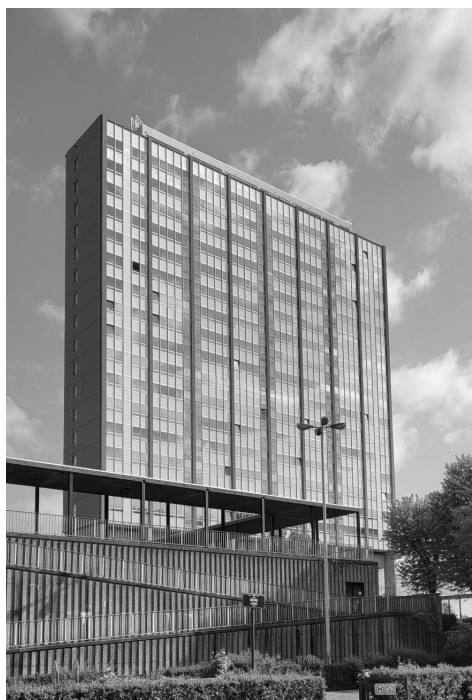
Fig. 18. South facade of the newly renovated Tower II; SLRB 2023.
