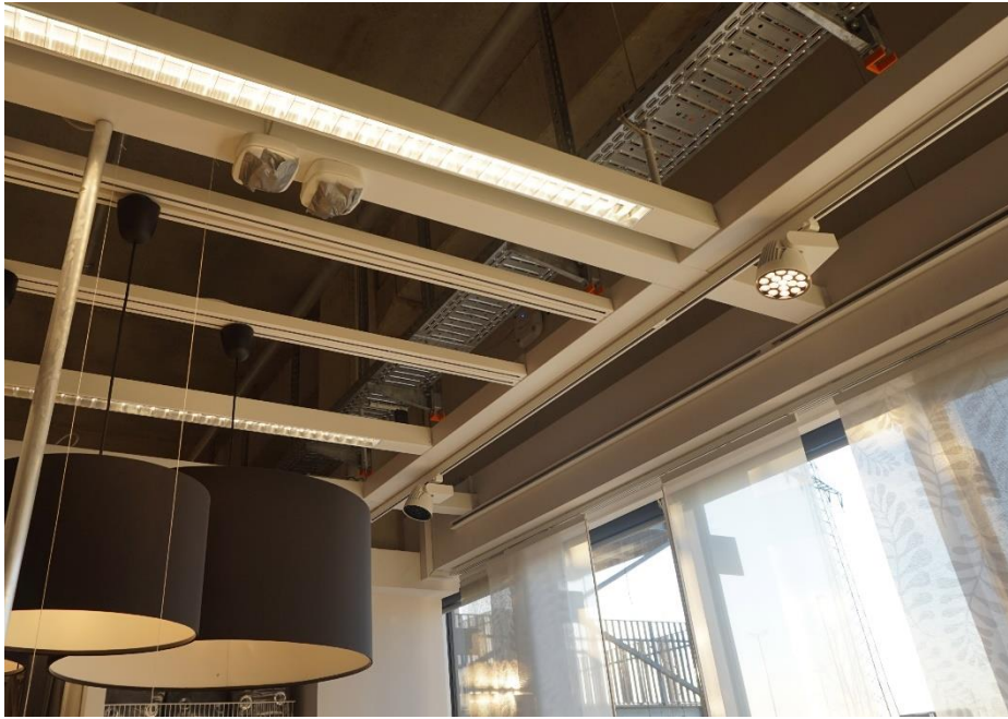
283 Figure 4. Taped photosensors for DLCs were observed in some case studies. This was linked to unwanted 284 fluctuations in light levels, due to either direct reflections from venetian blinds to the photosensor, or 285 changes in surface reflectance within the room. Source: Lund University.
