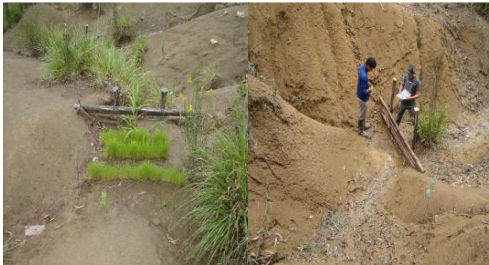
Figure 8: Construction of check dams in the active gully channels of the micro-catchments AI and DI (photo: Pablo Borja, 2012).
