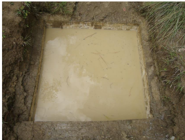
Figure 27: An example of a sediment trap that was constructed at the outlet of the micro-catchment to estimate the sediment export.
