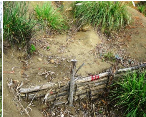
d) wooden dams for sediment control
