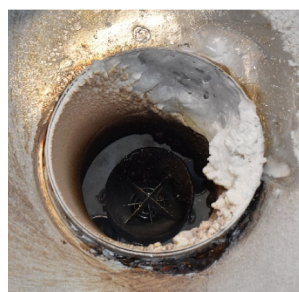
(c) The hot air distribution chamber
